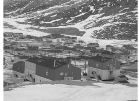
The CENTRON Meters were installed on house exteriors with no protection from winds, rain, snow, and sand dust.
