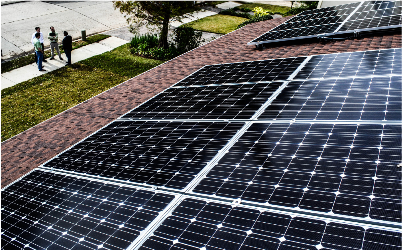
PosiGen Rooftop Photovoltaic Installation
