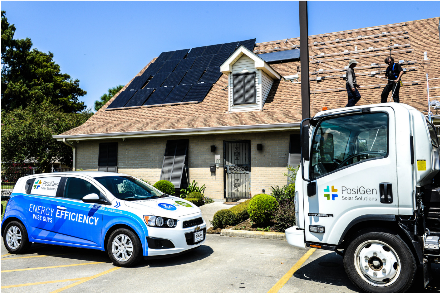
PosiGen Installation Team at Customer Premise
