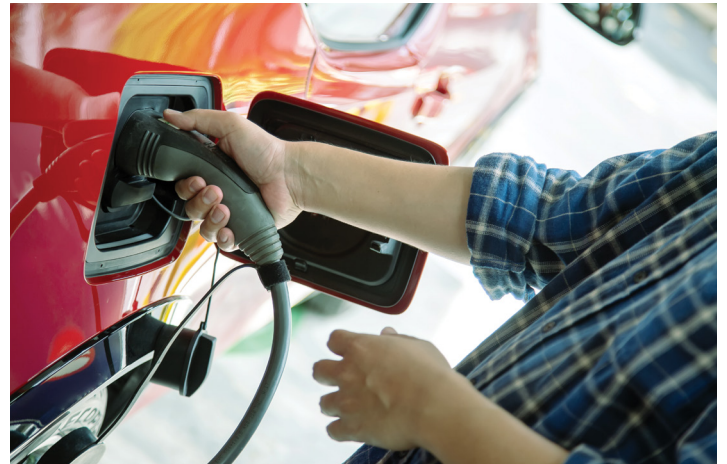
Thousands of electric car chargers are being fast-tracked to connect to the electricity network in the South East
